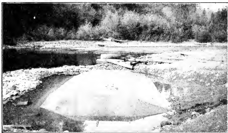
FIG. 5.—CONCRETE SUPPORT FOR TRIANGLES, FIRST UNIT, ANCHORAGE BLOCK IN BACKGROUND.
